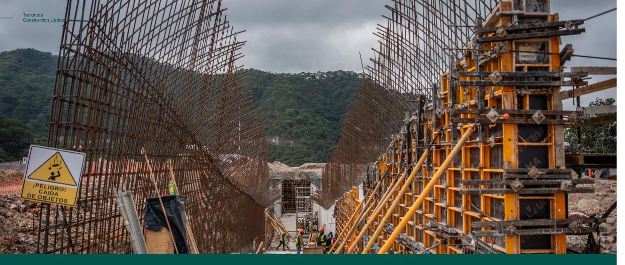
Coarse Ore Stockpile & Reclaim Area Rebar installation and forms for the coarse-ore stockpile reclaim tunnel (COSRT).
