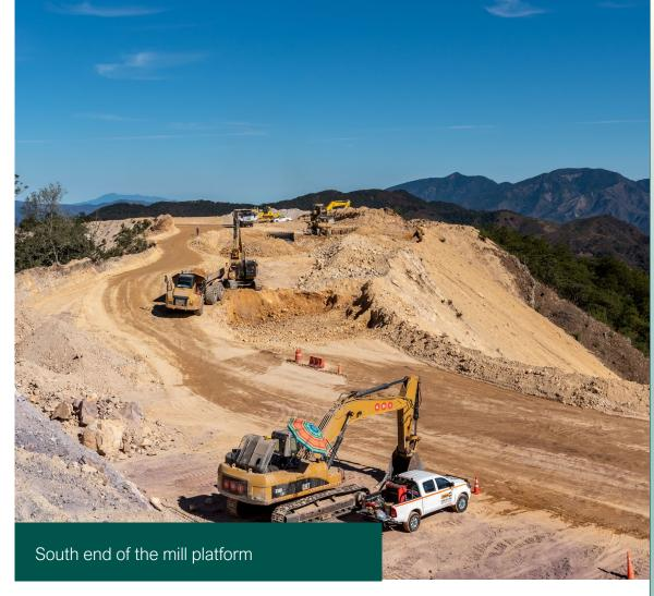
Over 250,000 m<sup>3</sup> of material has been removed to create a platform for the mill, which has a small footprint. Concrete work is planned to start before the onset of the rainy season.
