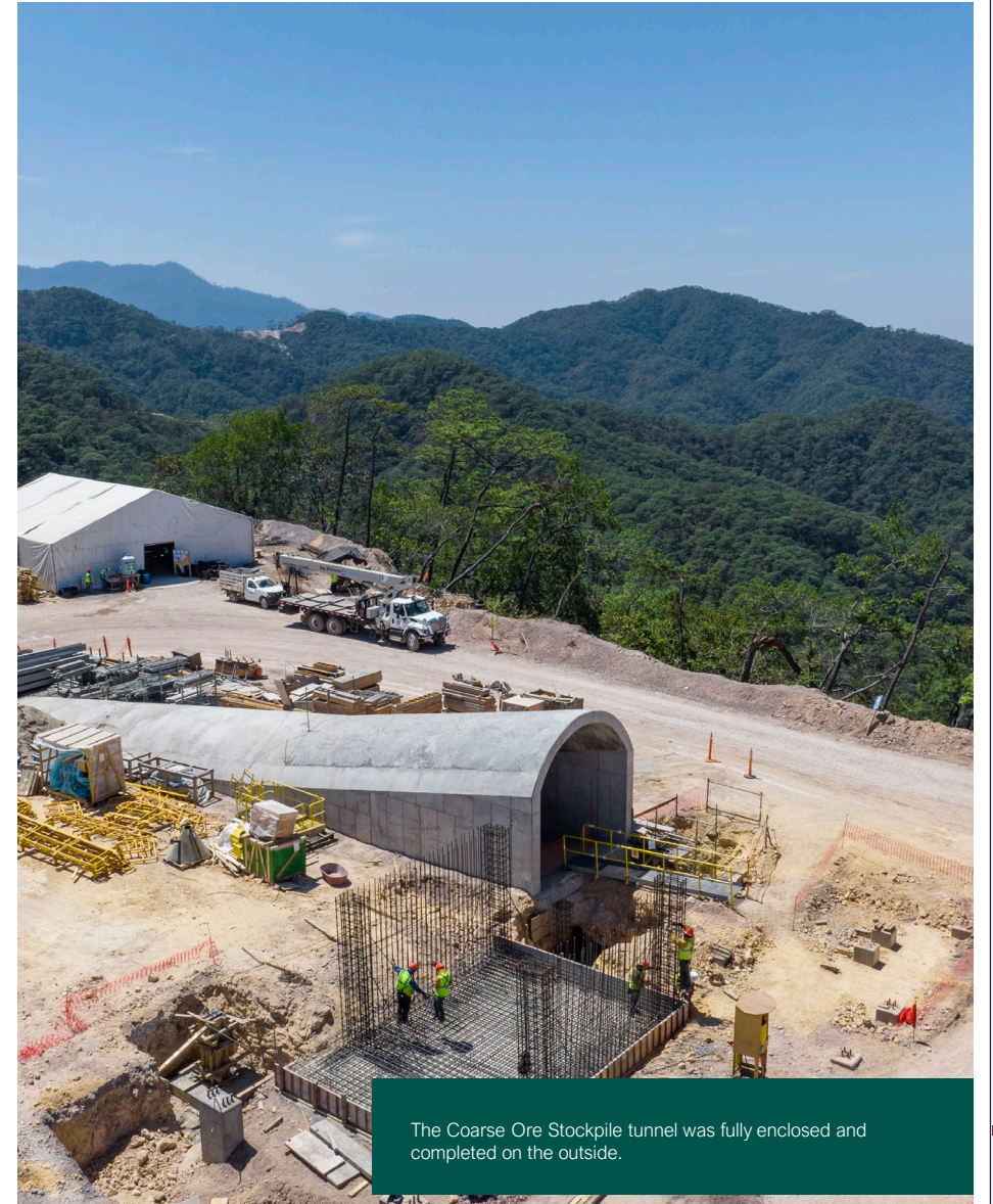
Excavation continues in the TSF embankment area and Lower Platform to allow for concrete work to start in Q2.
