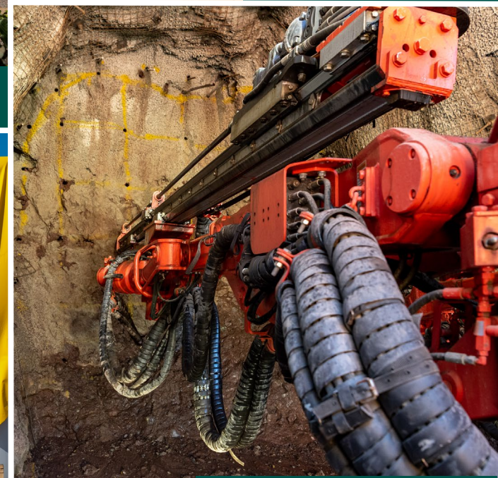
Mine development advances at Portal 2 & 4
