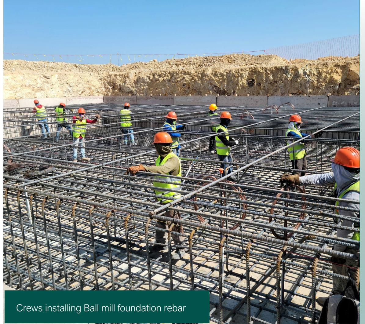
Crews installing Ball mill foundation rebar
