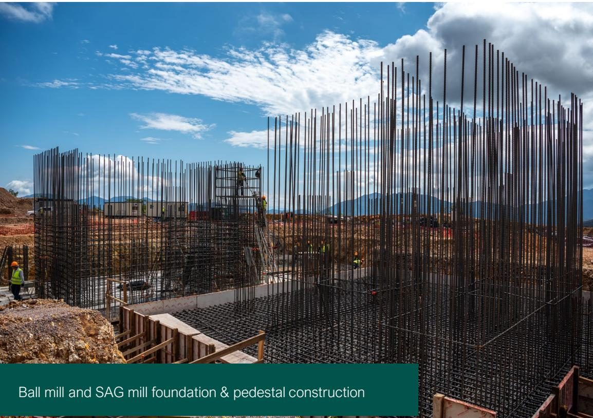
Ball mill and SAG mill foundation & pedestal construction
