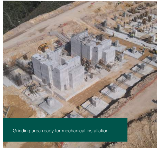
Grinding area concrete nearly complete
