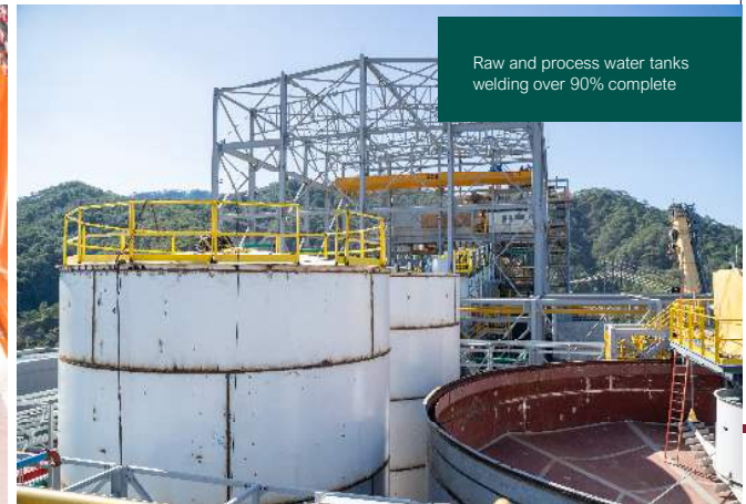
Lower Platform and TSF Area
