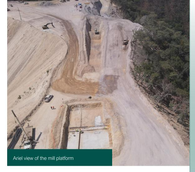
The plant site is a priority infrastructure area where leveling and grading for drainage is complete.
