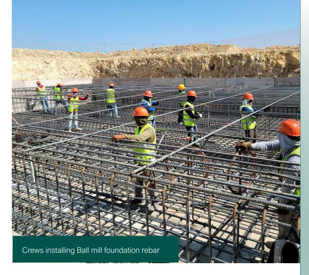
Rebar installation prior to the continuous Ball mill foundation pour.
