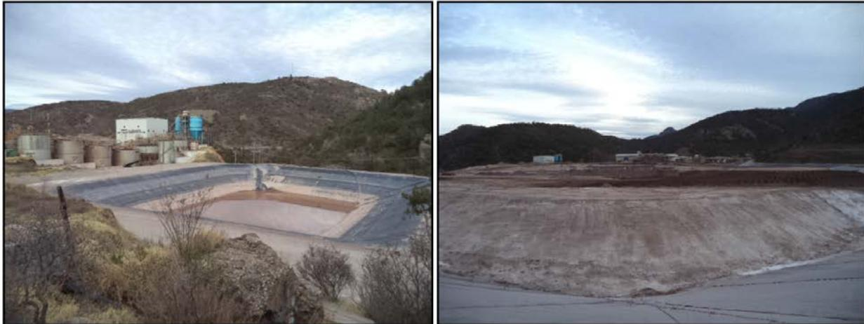
Figure 18-4 View of the new Rosario Tailings Water Pond with Capacity 10,000 m<sup>3</sup> (on the left); View of the Dry Stack Tailings Dam from the Northwest to Southeast (on the right)
