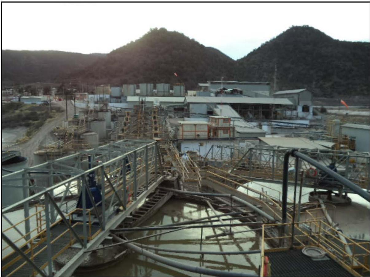
Figure 17-1 View of Leach Tanks and CCD Circuits
